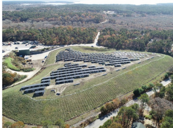
Solar panels on capped landfill, Photo courtesy of Wellfleet Energy and Climate Action
