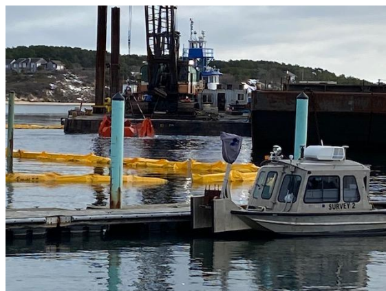
Dredging in the Wellfleet inner harbor
