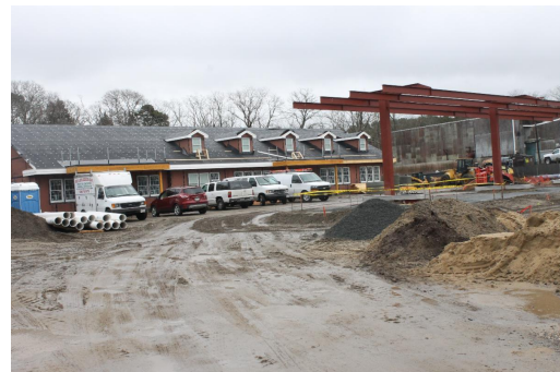
Cumberland Farms Construction, early February
