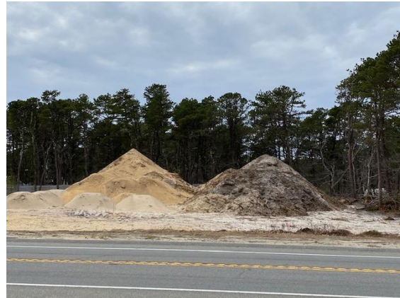
Old Wharf Rd and Route 6 after clearing
